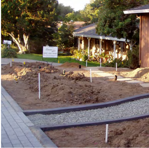
Soil Excavated from Walkway used for Mound
