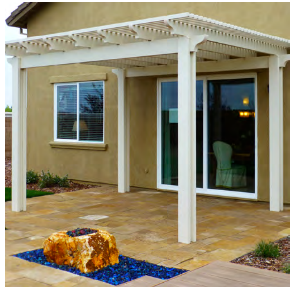
Overhead Structure & Deck Made of Composite Materials
