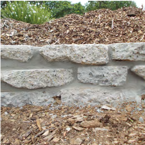
Close-Up View of Wall
