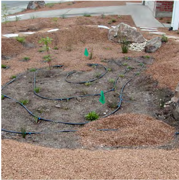
Rain Garden with Low-Volume Drip Emitters during Construction
