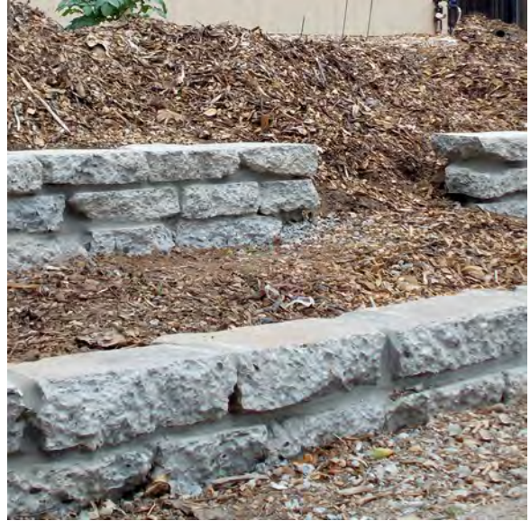
Planting Beds during Construction
