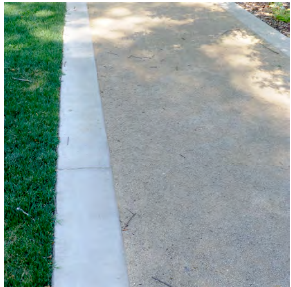
Decomposed Granite (D.G.) Path with Concrete Edging
