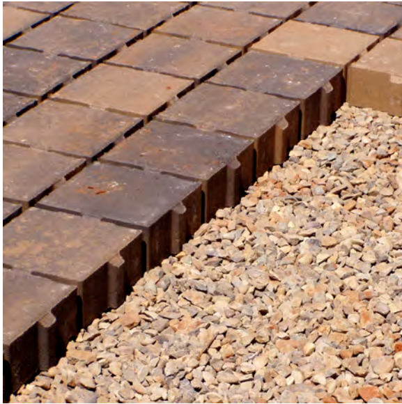
Walkway during Construction www.basalite.com
