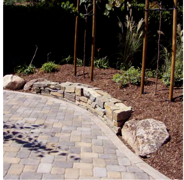
Permeable Walkway and Seal Wall Retaining Mounding Soil
