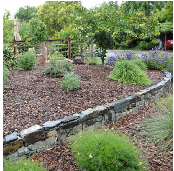
Raised Planting Bed with Mounding Soil Retained by Ledge Stone
