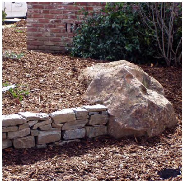
Dry Stack Natural Stone Wall with Moss Rock Boulder
