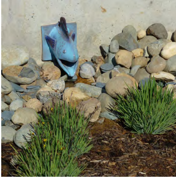
Elk Grove Rain Garden Drainspout
