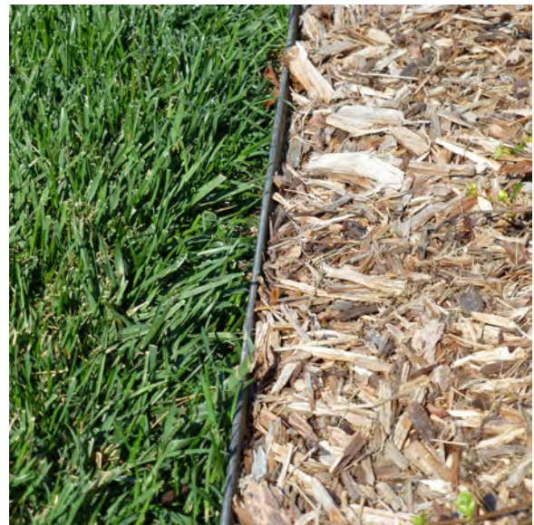
Metal Edging between Turf and Walk-On Mulch
