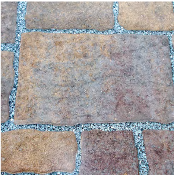
Pavers with Rock in Joints for Permeability
