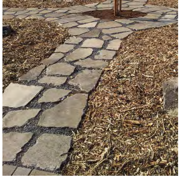
Permeable Recycled Concrete Path
