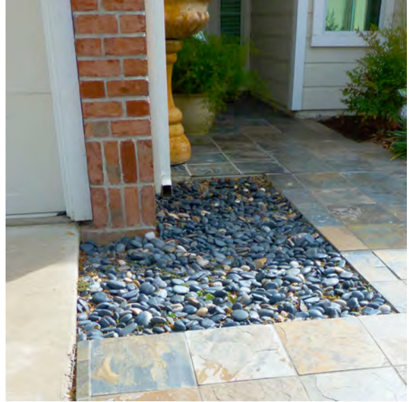
Downspout Directed to Permeable Cobble
