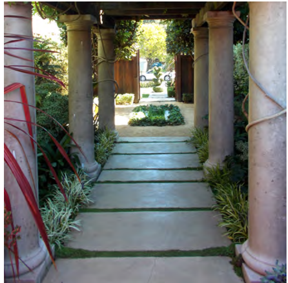
Concrete Sections with Groundcover in Joints
