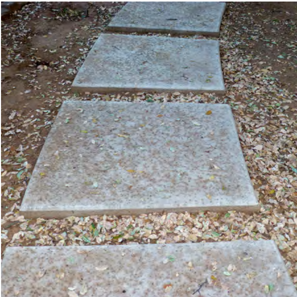
Concrete Sections with Leaf Mulch
