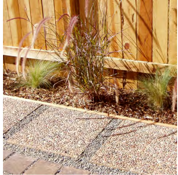
24" x 24" Exposed Aggregate Pavers with Rock in Joints
