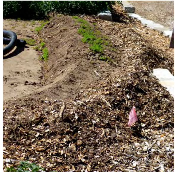
Soil Excavated from Rain Garden used for Mound during Construction
