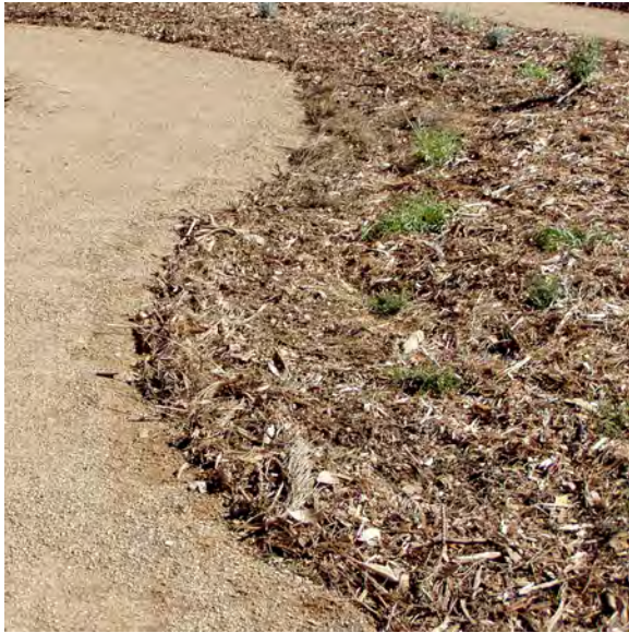
Decomposed Granite (D.G.) Path with Mulch
