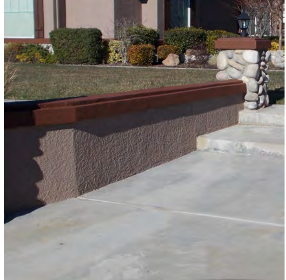
Stucco Seat Wall
