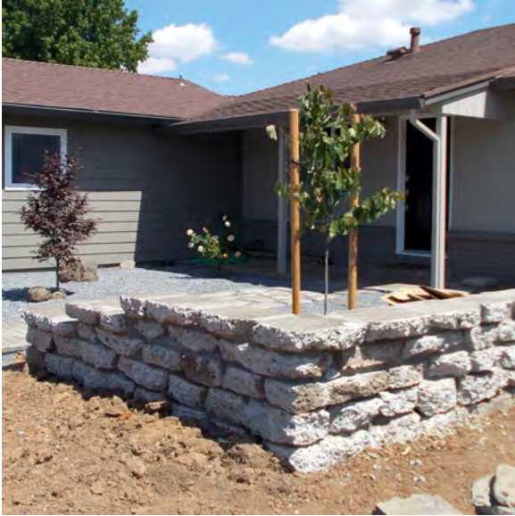
Wall During Construction
