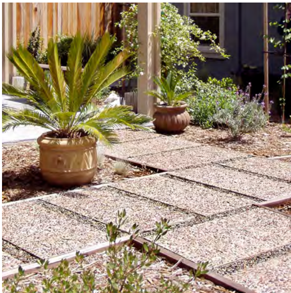
18" x 36" Exposed Aggregate Paver Installation
