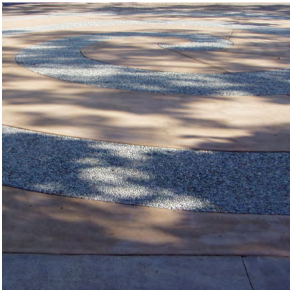
Permeable and Non-Permeable Concrete
