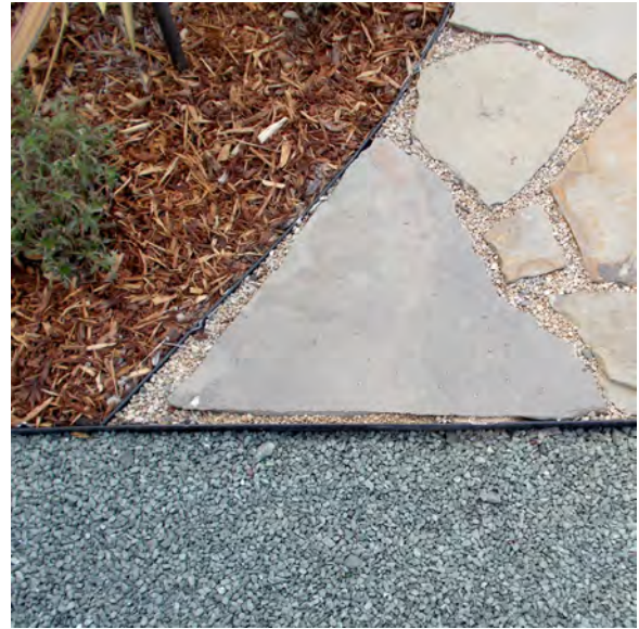
Metal Edging with Flagstone, Mulch, and D.G.
