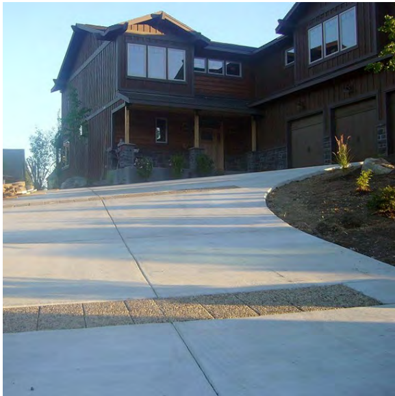
Installed Across Driveway
