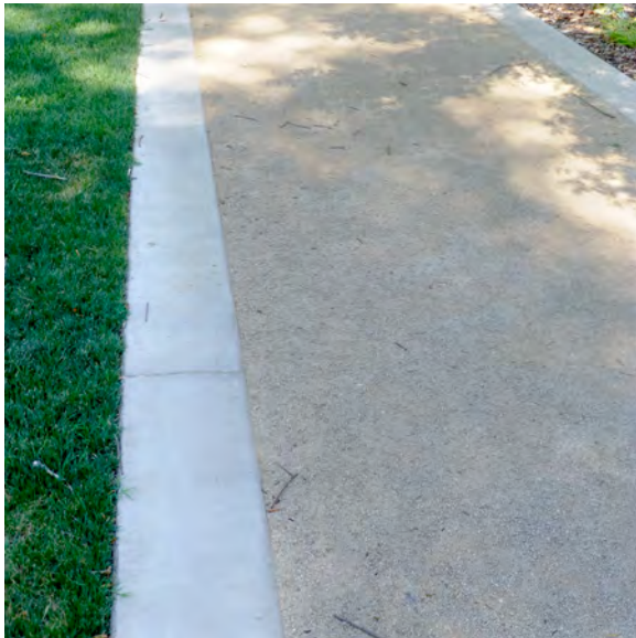
D.G. Path with Concrete Edging
